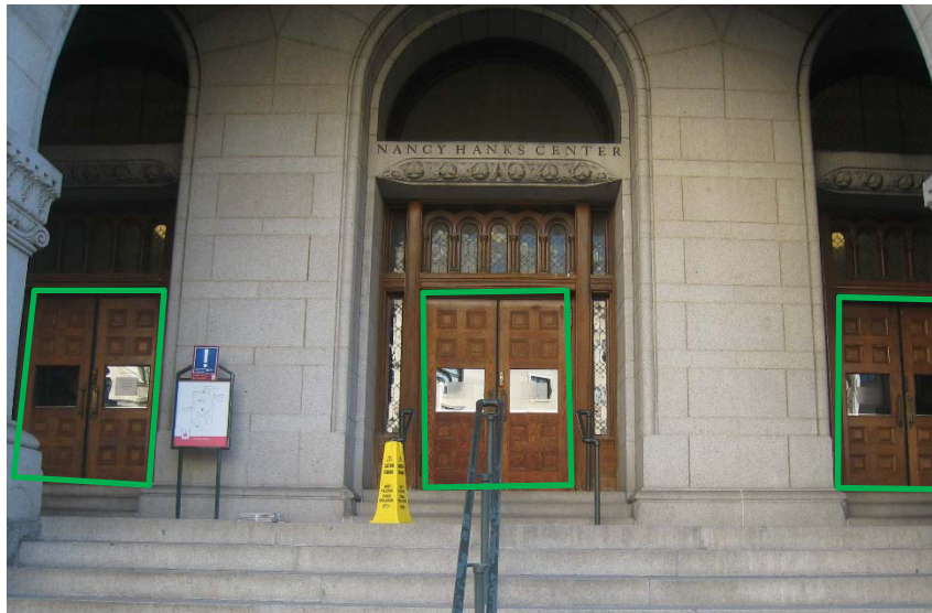
Existing portion of wood door set to be replaced with glass
